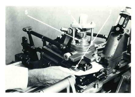
well be thought, but by the action of the centring pin loading spring (6), in which the upper end of the centring pin is seated. The descent of the matrix lifter lever (15) presses the centring pin loading spring upon the coupling head (1), beneath which is located the centring pin guide spring which terminates on the matrix lifter (3).
